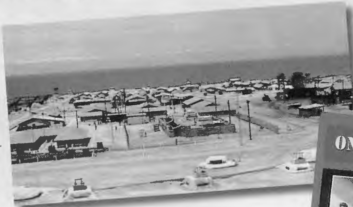
CCN in Da Nang, facing east toward the South China Sea. Photo: Author
